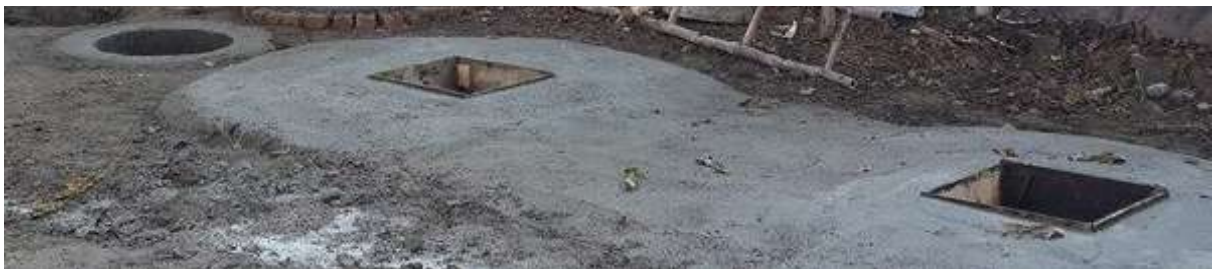
Picture 2, Small Biological sewage treatment plants consists of three well
