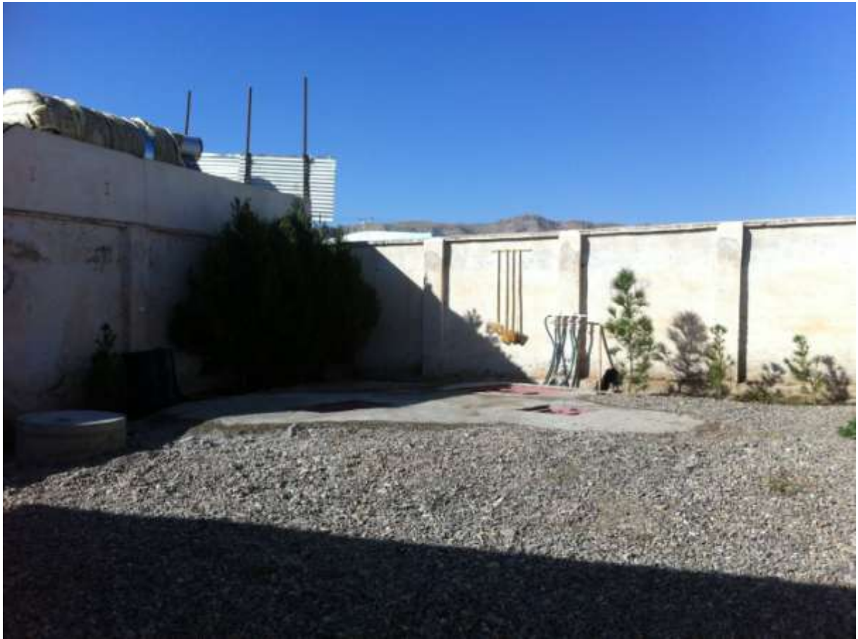
Picture 7 , The Biological sewage treatment plants, (Herat, Family center, for 100 -120 people)
