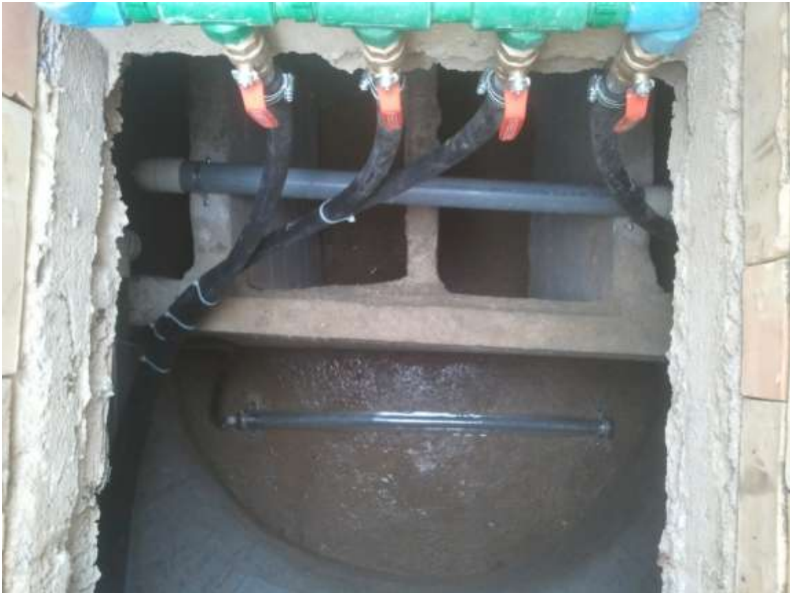
Picture 3 , First well, the Aerob part of system, where is installed the air element
