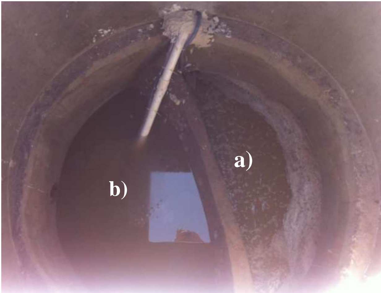
Picture 5 , Second well a) The biological filtration and purification of system, b) The water after filtration and purification
