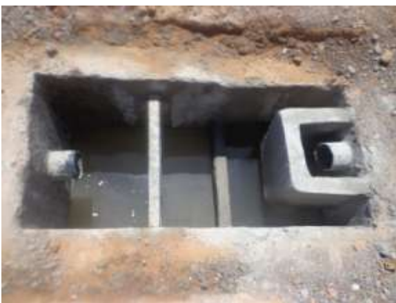
Picture 12, The Sewage water and fat water treatment system in Shikiban vilage of Zindagan district of Herat province (for 100 to 120 people) - The using of water after purification and filtration for agriculture
